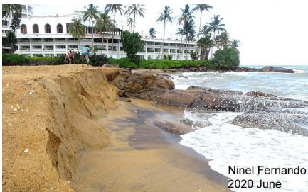
Figure 2: Shows the height of the sand deposited that would have covered the rocks at right as well as the bay behind.
